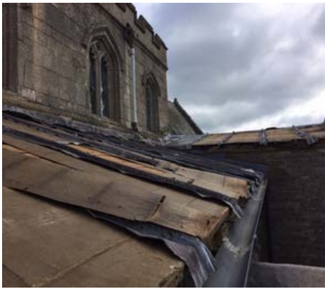
South Aisle roof repair: Condition following lead theft and the completed roof repair
