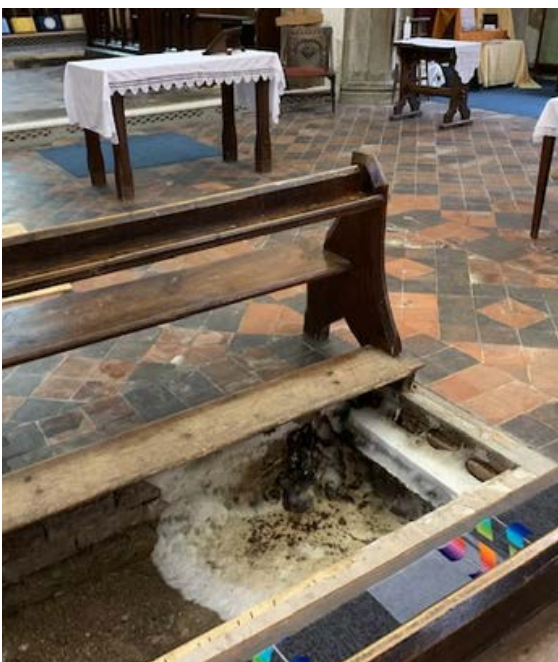
A dry rot outbreak beneath a pew platform due to inadequate underfloor ventilation to the floor void
