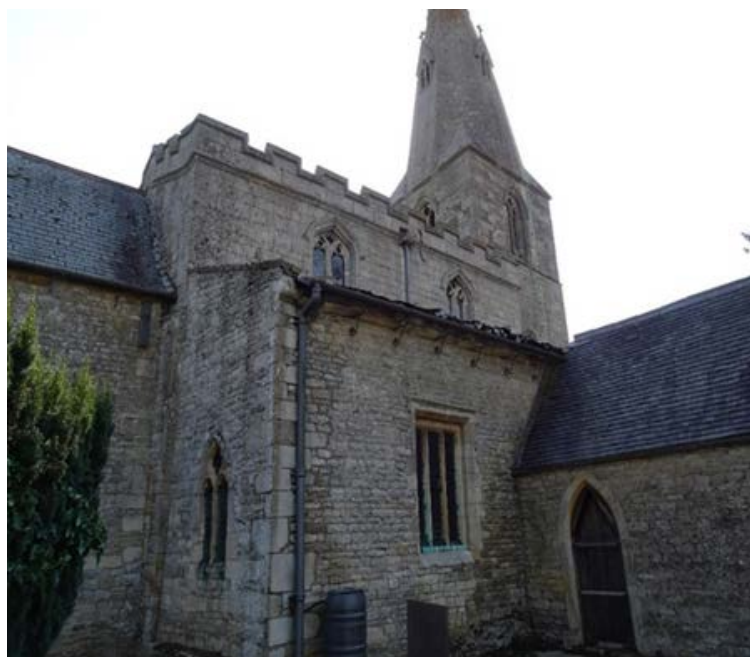
Gutters and Downpipes Repaired or Replaced and Gable and Clerestory pointed
