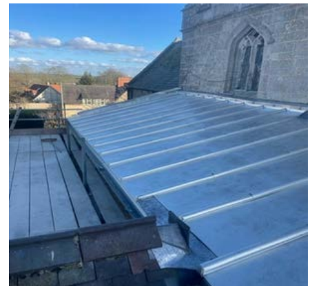
North Aisle roof repair: Condition following lead theft and the completed roof repair
