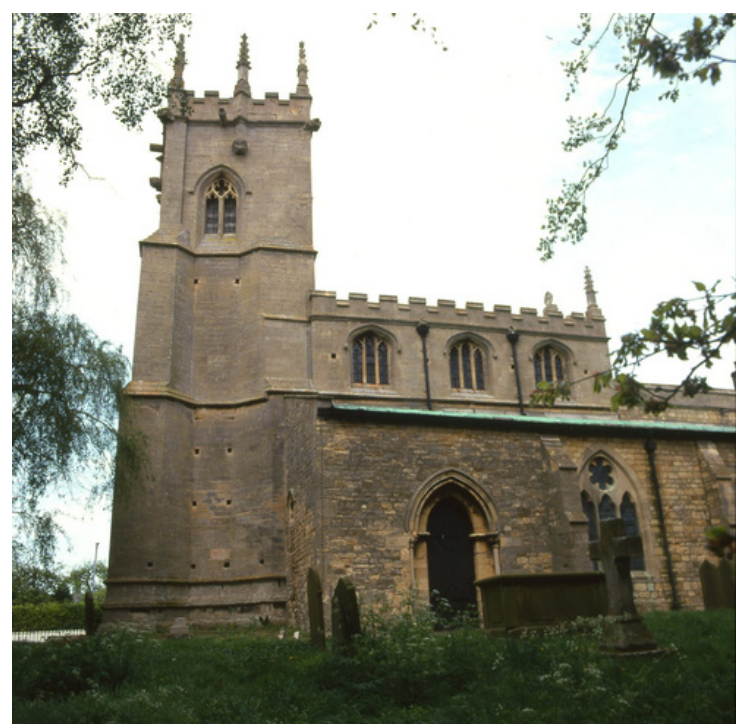
Fiskerton, St Clement with clear putlog holes in tower and clerestory level
