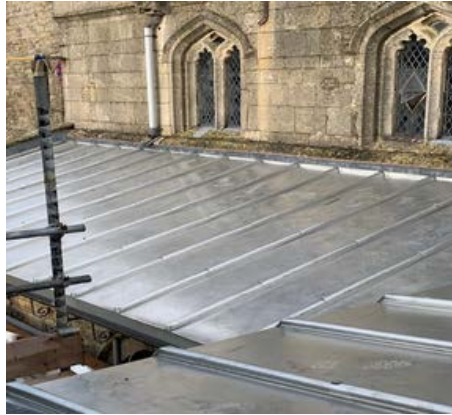
South Aisle roof repair: Condition following lead theft and the completed roof repair
