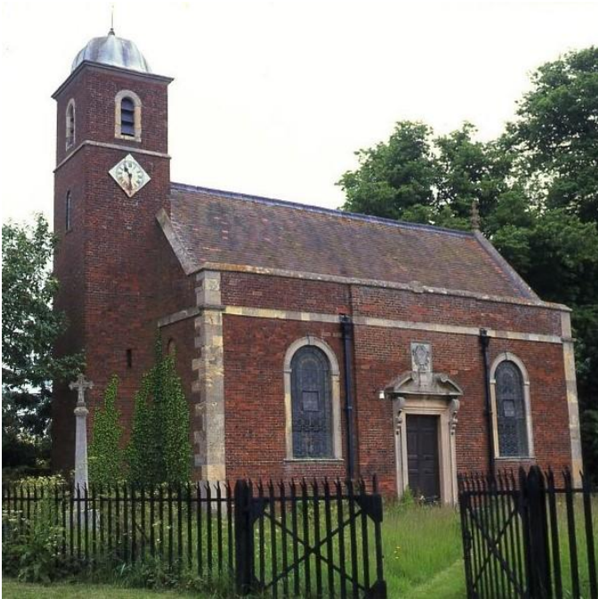
Left Stainfield St Andrew an early Georgian church built from brick with dressed stone details.
